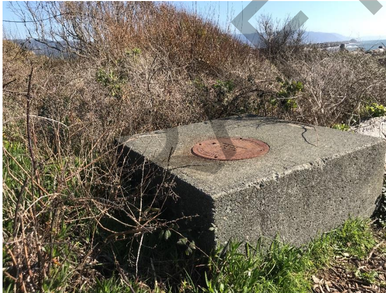
Feature 8, Gravity manhole in good condition.
