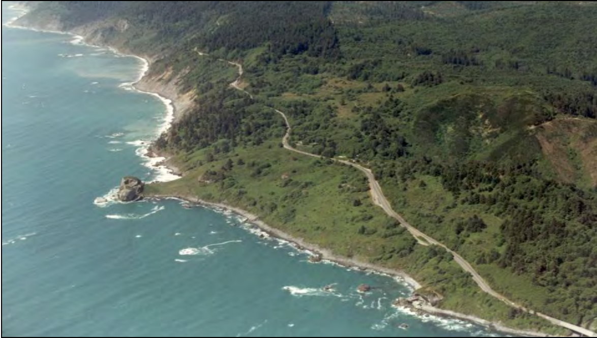
Figure 14-6. Highway 101, Last Chance Grade
